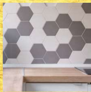
DADO CERAMIC TILES 600 MM ABOVE THE COUNTER
