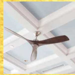
CEILING OIL BOUND DISTEMPER
