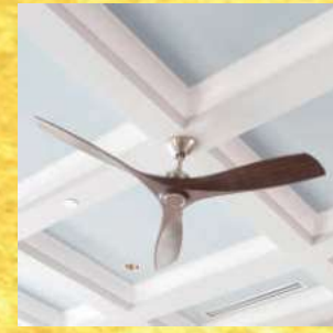
CEILING OIL BOUND DISTEMPER
